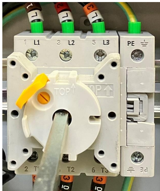
Figure 7 - Electrical connection of the machine
